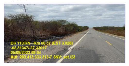
According to DNIT (2006b) and Rodrigues et al. (2008), the incidence of slips on the edge of the pavement may occur due to some factors, such as: poor dosage of the asphalt mixture; excess binder, generating high humidity from the coating to the lower layers; inadequate compaction of the asphalt mixtures or the upper portion of the base layer, and plastic deformation of the coating due to the influence of high temperatures.
