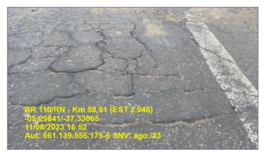
The appearance of cracks in block shapes occurs as a result, according to DNIT (2005) and Rodrigues et al. (2008), of the following aspects: contraction of the coating material, due to temperature variation; considerable loss of the characteristics of the asphalt binder; fragility in the tensile strength of the asphalt mixture; Union of transverse and longitudinal cracks in cement-based coatings.
