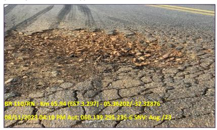
Figure 6 shows that pathologies do not always occur in isolation, because traffic, together with the action of other triggering agents, such as rainwater, initiates the disintegration of part of the coating forming the pans and, thus, promotes surface irregularities and, with the increase in traffic intensity in the first irregularities, results in a chain of effects.
