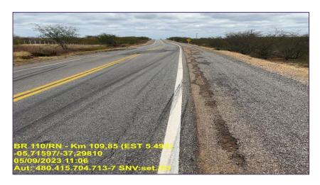
According to DNIT (2005) and Rodrigues et al. (2008), the appearance of these longitudinal cracks occurs due to these factors, such as: poorly executed construction joint; inadequate connection between the layers launched in sequence to form traffic lanes; emergence of settlements in the layers below the coating; contraction or expansion of the coating due to the technical gradient, or aging of the asphalt, and concentration of stresses in the vicinity where the crack manifested.
