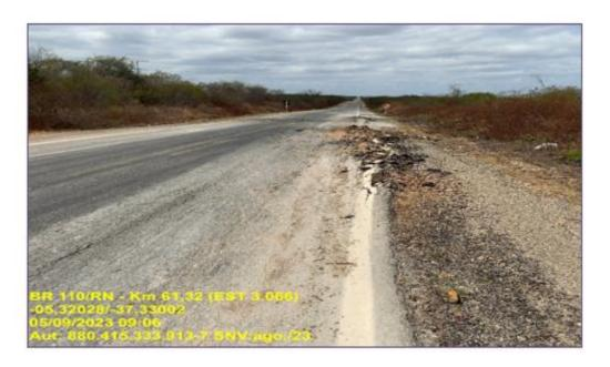
Plastic sinkings are identified by depressions on the surface of the pavement, and can be generated due to some aspects, such as: plastic deformation of the upper and/or adjacent layer, which can even affect the subgrade; excessive action of traffic loads; poor soil compaction, and deficiency in the dosage of the asphalt mixture (Bernucci et al. (2008); DNIT, 2006b; SILVA, 2008).
