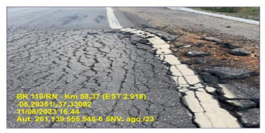
According to DNIT (2005) and Rodrigues et al. (2008), the interconnected cracks that hold the appearance of alligator leather arise due to some factors, such as: contraction of the asphalt layer due to temperature variation; the material that constitutes the coating has low viscosity; constant deformations caused by traffic loads, and low thickness of the coating layer.
