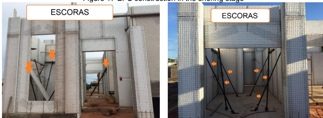
Figure 17 EPS construction in the shoring stage
