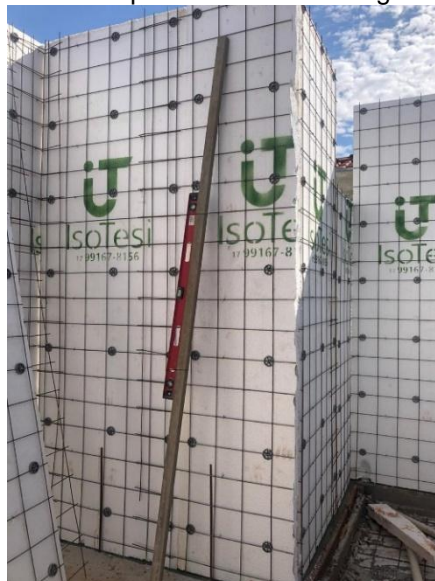
Figure 22 Use of the plumb bob for leveling the EPS panel
