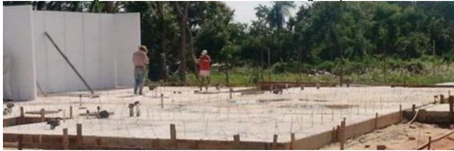
Figure 15 – Starts on the radier for fixing the panels
