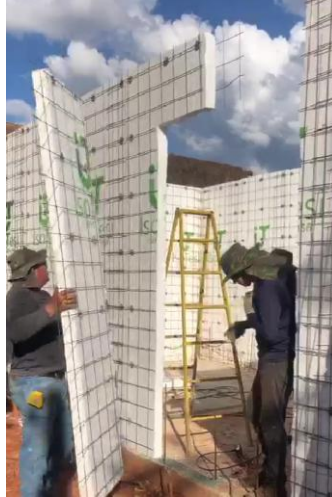
Figure 21 Opening frames in the EPS panel
