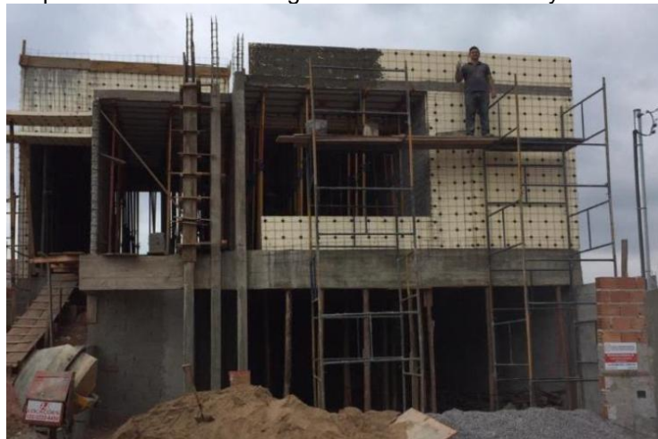
Figure 2 Example of construction using the EPS construction system in Varginha/MG
