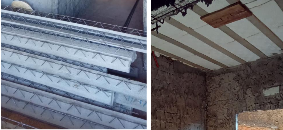
Figure 29 Lattice slab rails (left) and completion of the one-room slab (right)
