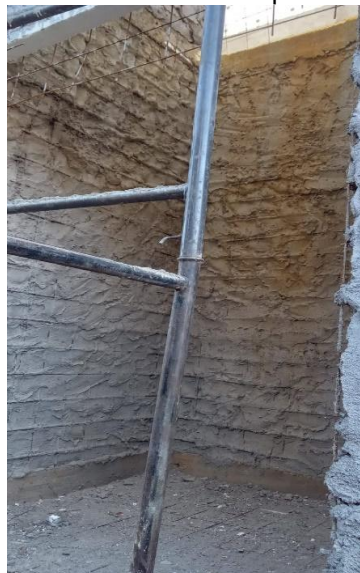
Figure 28 Elevator shaft in the plastering phase
