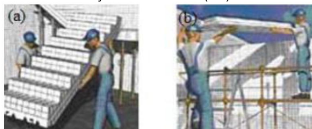
Figure 18 – Assembly of the staircase (left) and the slab (right)
