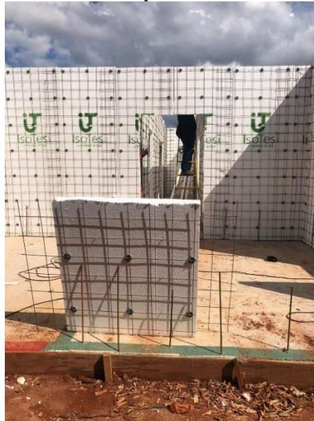
Figure 19 – Radier already concreted and color marking
