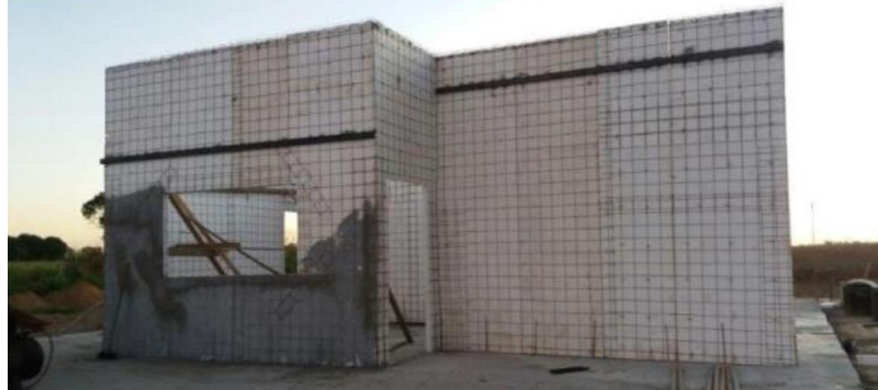
Figure 1 Example of construction using the EPS construction system
