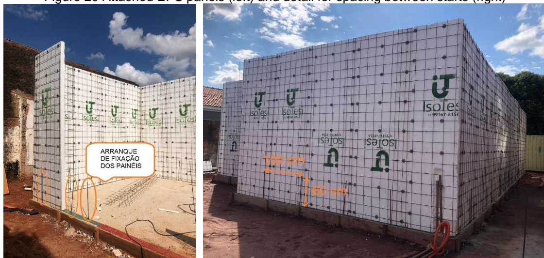
Figure 20 Attached EPS panels (left) and detail for spacing between starts (right)
