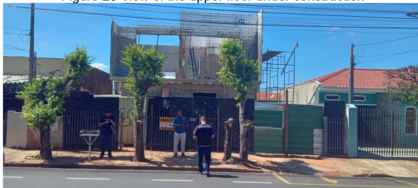
Figure 26 View of the upper floor under construction
