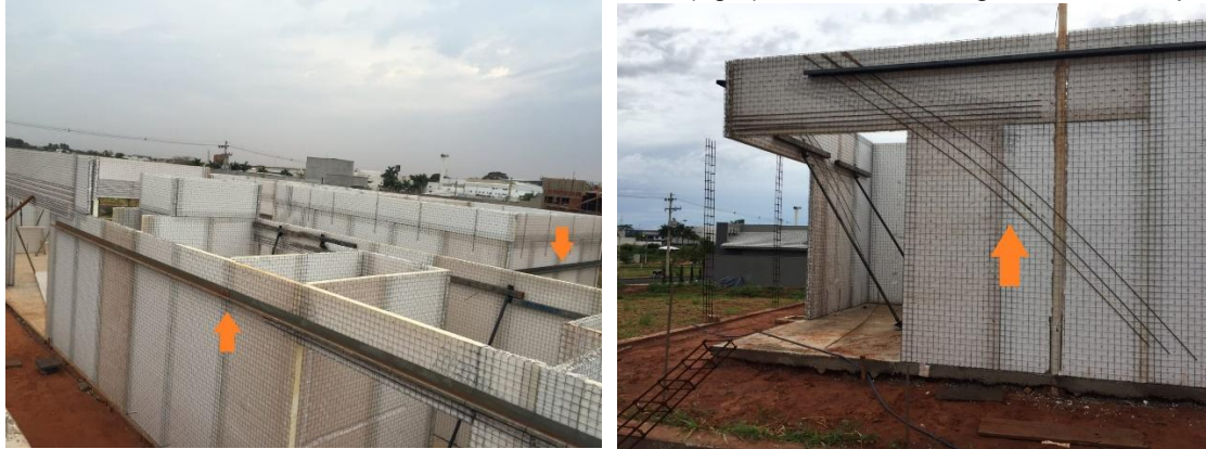
Figure 18 \u2012 Use of metal stringers (left) and steel rebar (right) for horizontal alignment of EPS panels
