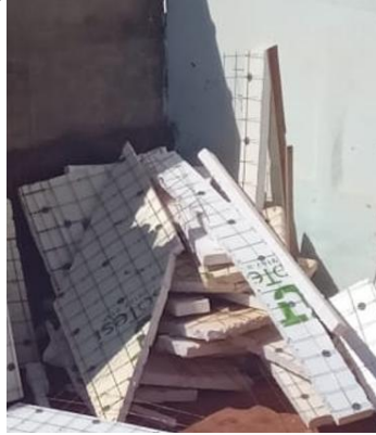
Figure 33 – Waste from EPS panels
