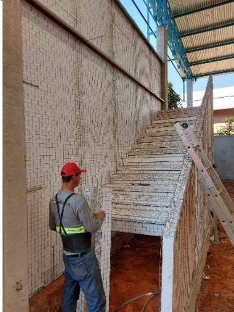
Figure 17 - Assembly of the staircase in EPS
