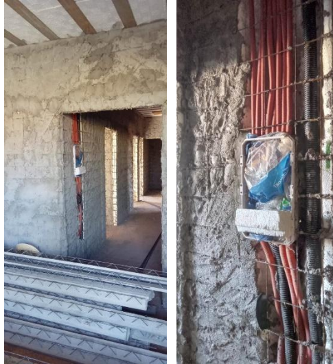
Figure 25 Detail of the switchboard attached to the panel in EPS
