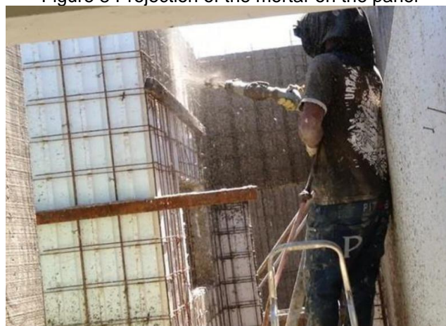
Figure 8 Projection of the mortar on the panel
