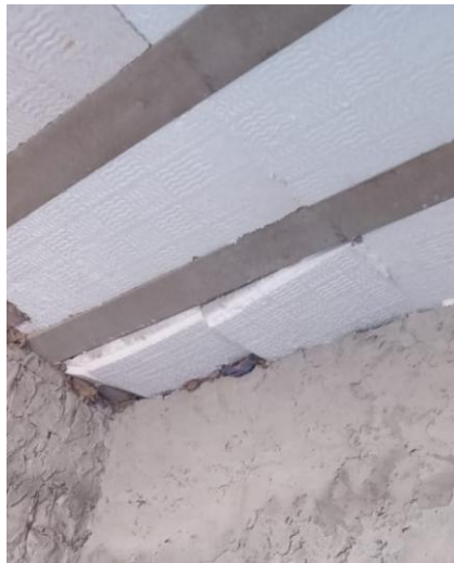
Figure 30 - EPS slab with concrete overhead at the corner of the slab
