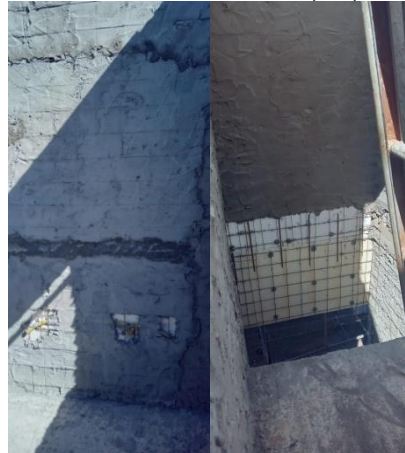
Figure 31 Plastering phase with structural mortar (left) and traditional mortar (right)
