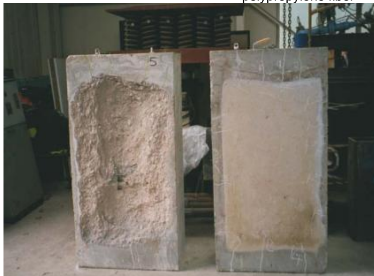
Figure 6 – Effect of delamination on fiberless concrete Fiberless concrete Concrete com 1000 g/m 3 polypropylene fiber
