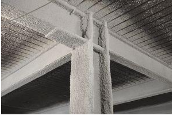
Figure 12 – Steel structure covered with fiber-reinforced mortar.
