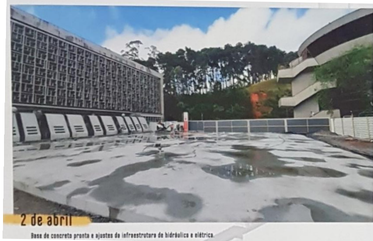
Figure 25 – Preparation of a shallow structure (radier) to receive the modules (04/02/2020)
