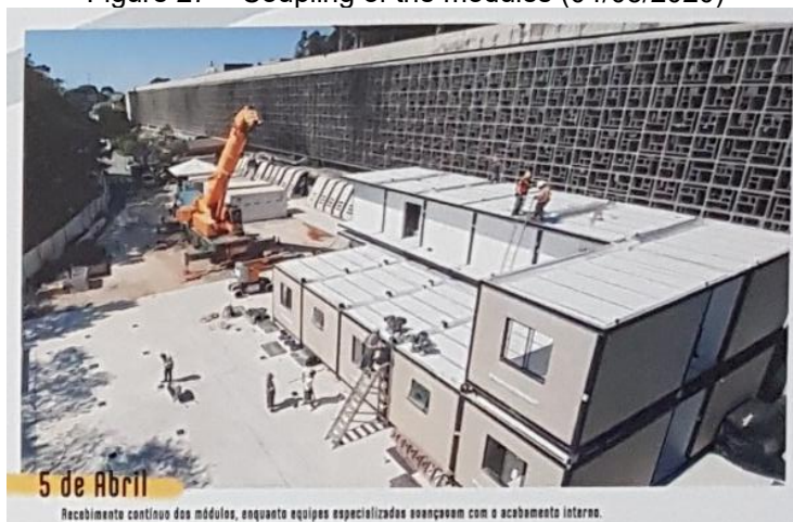
Figure 27 – Coupling of the modules (04/05/2020)
