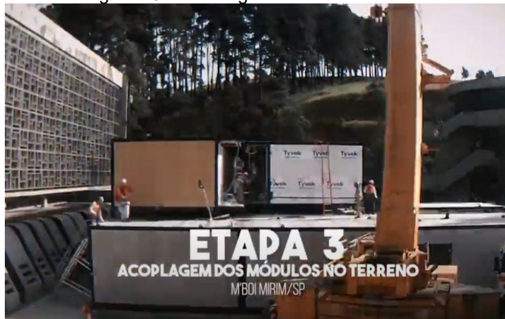
Figure 26 – Docking of the modules on site
