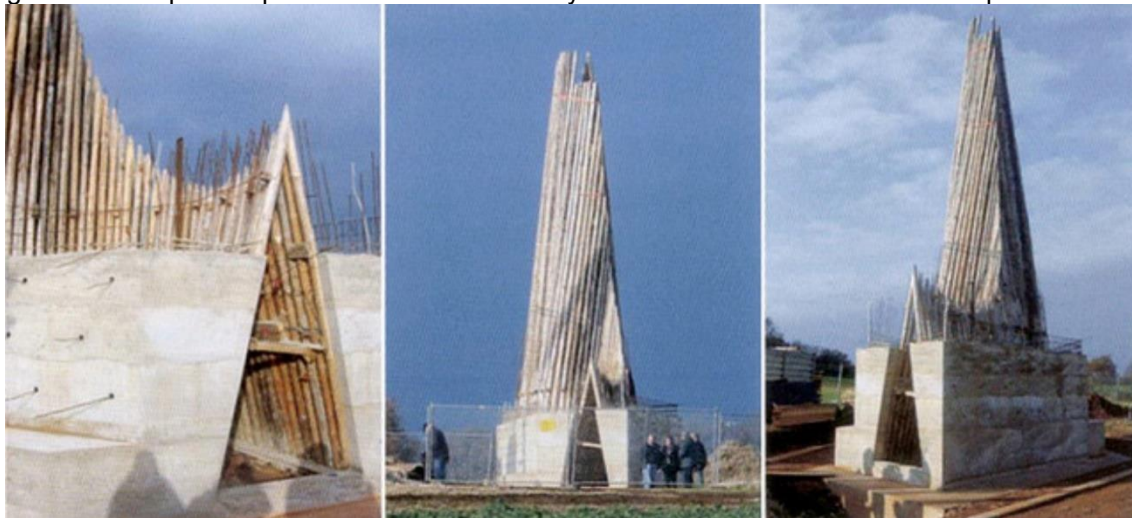
Figure 5 – Compaction process of the concrete layers between October 2005 and September 2006.
