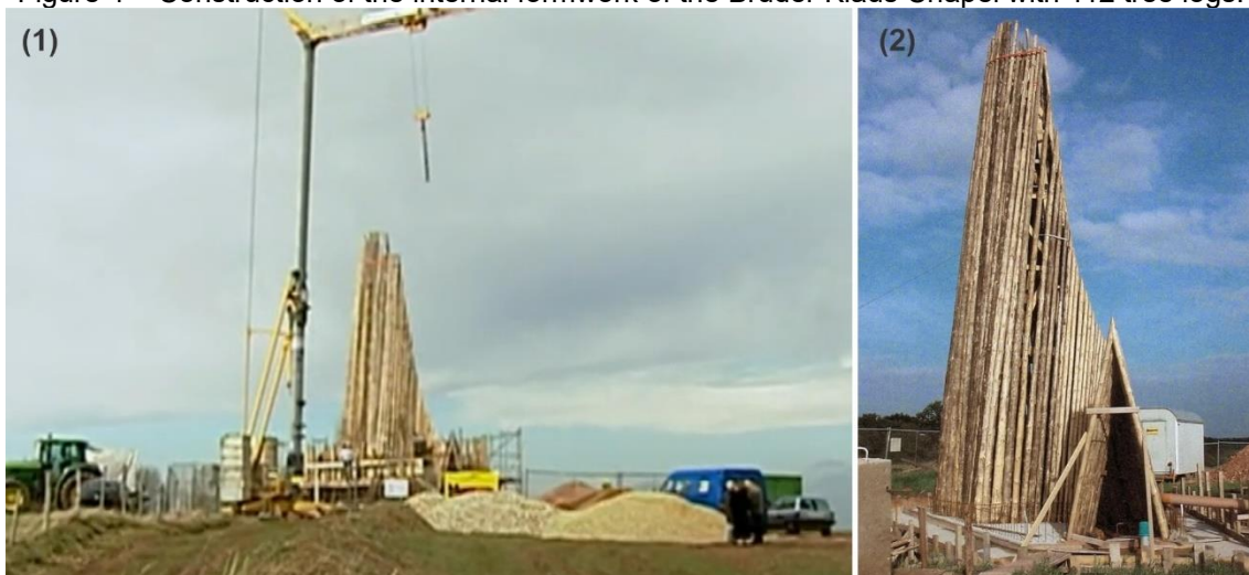
Figure 4 – Construction of the internal formwork of the Bruder Klaus Chapel with 112 tree logs.
