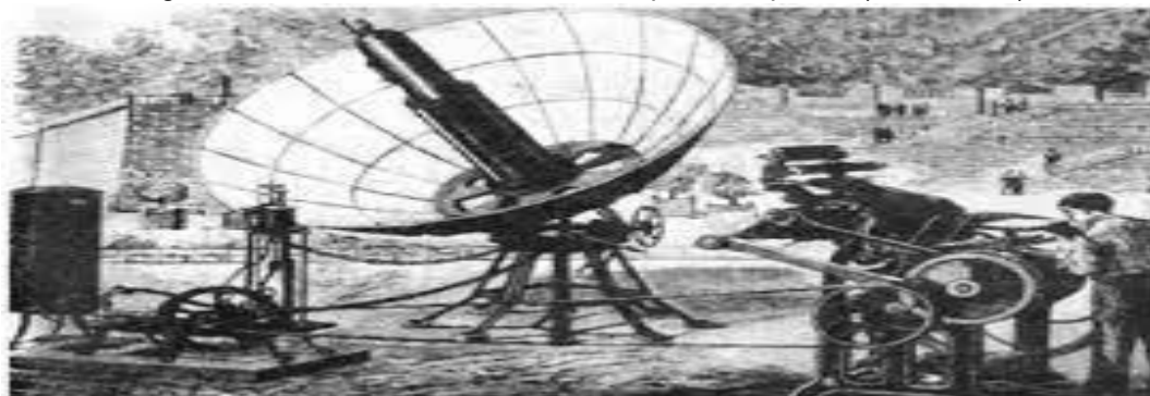
Figure 2 – Parabolic collector of a solar-powered printer (Paris, 1882)
