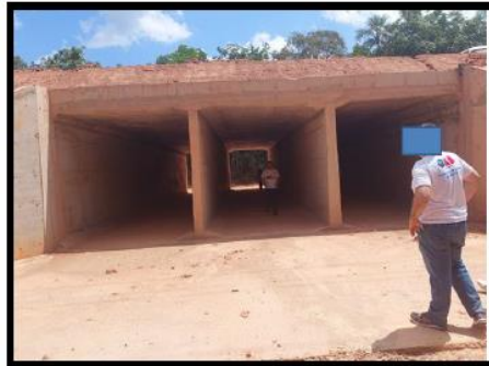
Figure 1. Fauna Passage located at Km 205 of BR-319 (Middle Section)
