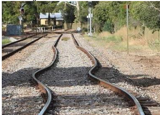
Figure 1: Surface Dilation in the rails
