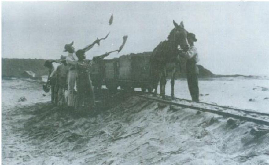
Figure 1 - Removal and transport of monazite sand from Guarapari in the early twentieth century.
