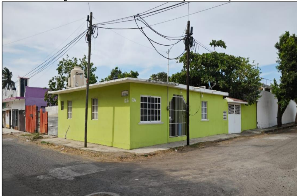
Figure 5. Construction of the case study in Veracruz port.
