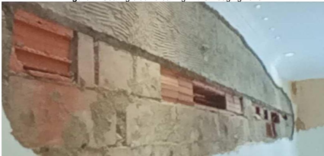
Figure 2: Sealing block breaking in the wedging zone.
