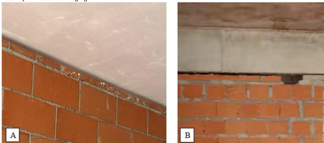
Figure 1: Opening between masonry and the slab (a). opening between masonry and beam (b). Both masonry will receive wedging.
