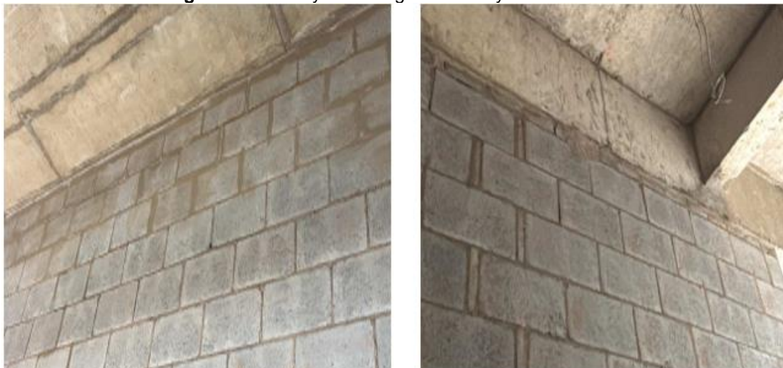
Figure 4: Masonry in sealing block ready to be finished.
