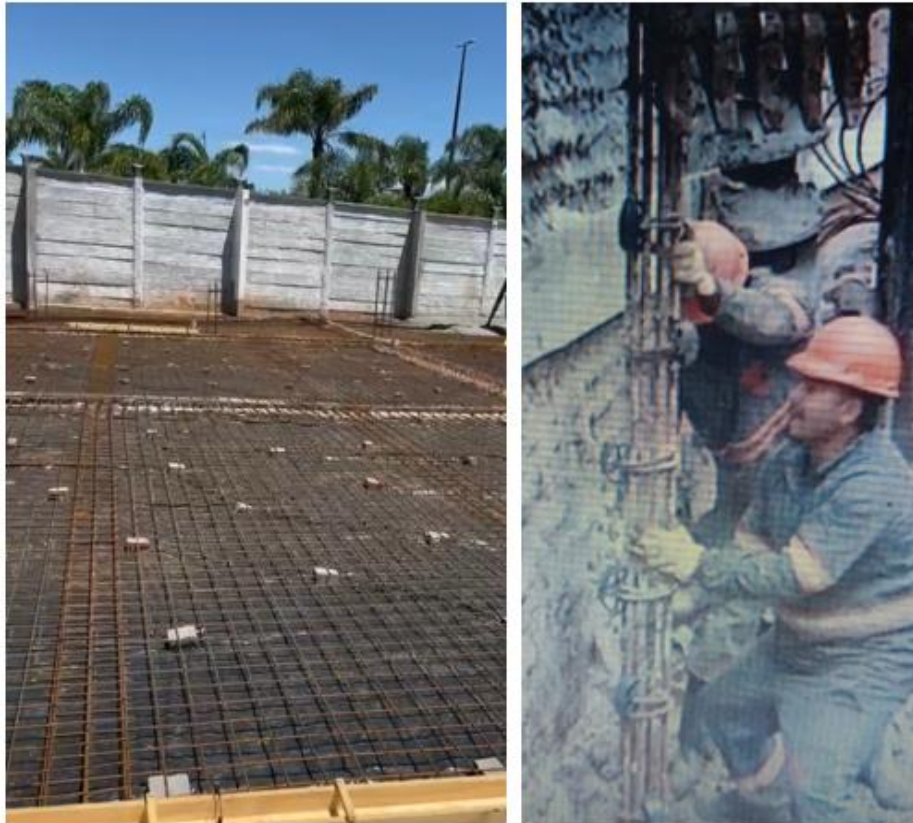
Figure 2 – Examples of foundation execution with spacers.
